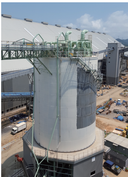
New Boryung thermal power Fly ash silo vent filter
